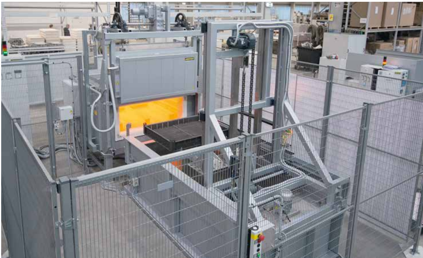
Fully automatic tempering plant comprising an annealing furnace, a water quench tank, and a two-axis manipulator
