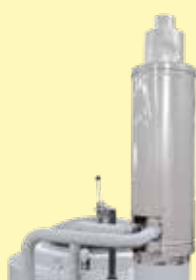
Heat exchanger in the exhaust gas duct
