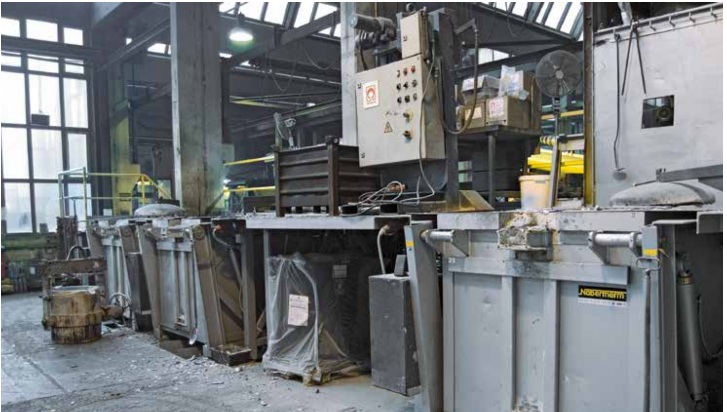
Three tilting furnaces with work platform for melting of aluminum
