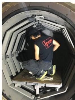
Insulation Overhaul
