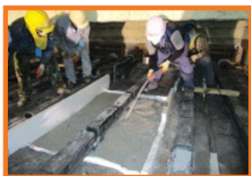
4. Lining (Refractory castable casting)
