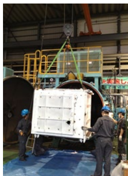
Overhaul of Hot Chamber
