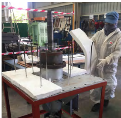
TAKE OLD INSULATION OUT AND INSTALL NEW ONE
