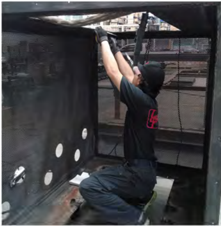
Taking off old insulation
