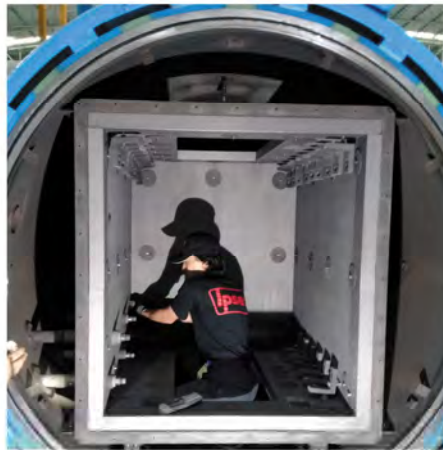
Changing insulation and heater
