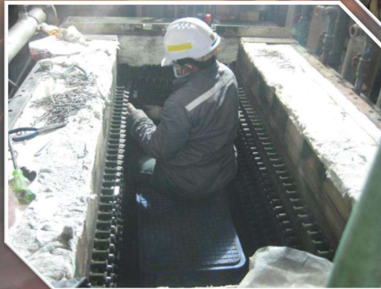
Repairation of Gas Generator
