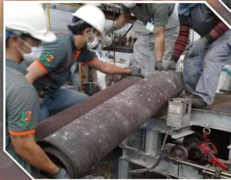
Installation of Mesh Belt
