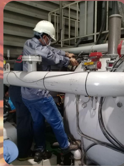
Helium leak testing and repair insulation in vacuum furnace
