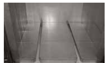
Track cutouts for pallet truck or charging cart
