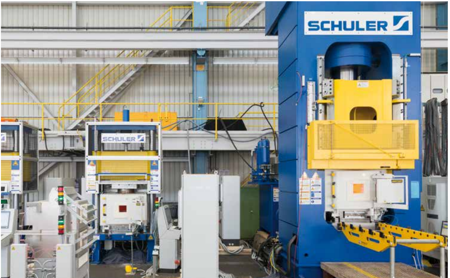
Furnace to preheat the press ram of a hot forging plant
