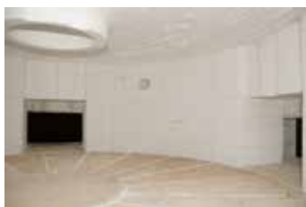
Rotary table with fire-resistant concrete plates to protect the insulation
