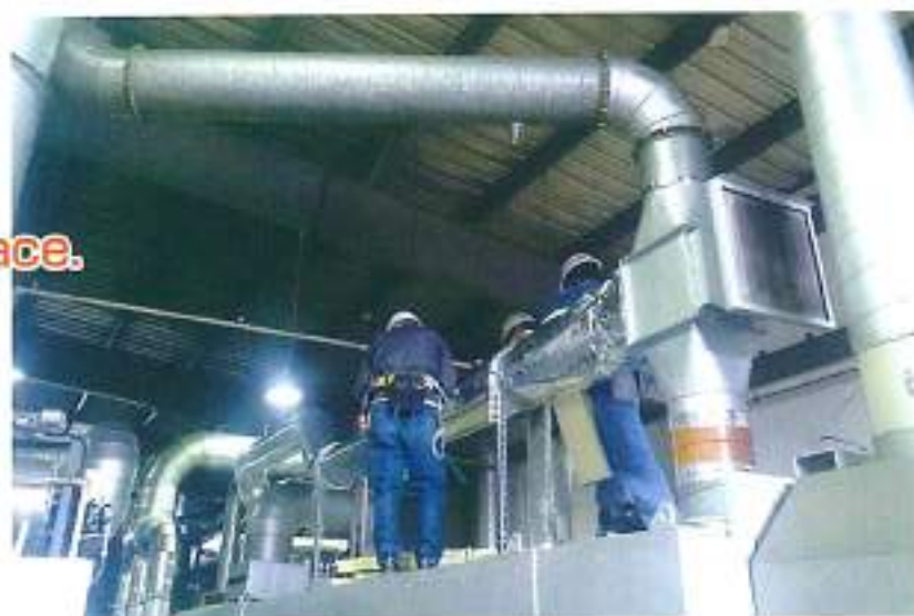
Installation work in Aichi prefecture. Installing to continuous painting drying furnace
